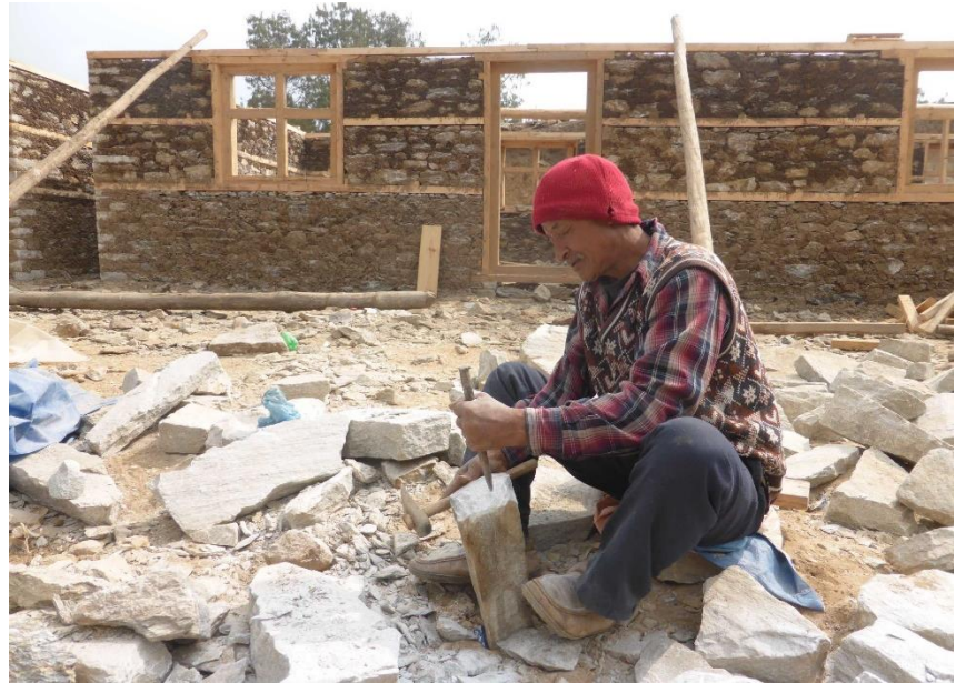
Corner stones and through stones are prepared and built properly for earthquake reinforcement
