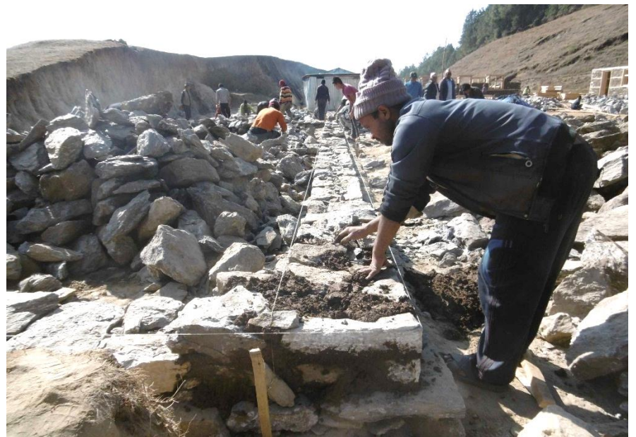
Foundations are done with big stones; all masonry work is done by hand
