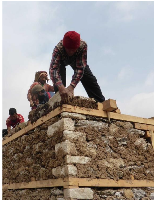
Corner stones and through stones are prepared and built properly for earthquake reinforcement
