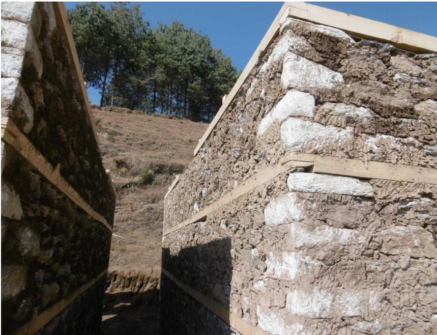
Corner stones and through stones are prepared and built properly for earthquake reinforcement
