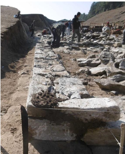
Foundations are done with big stones; all masonry work is done by hand
