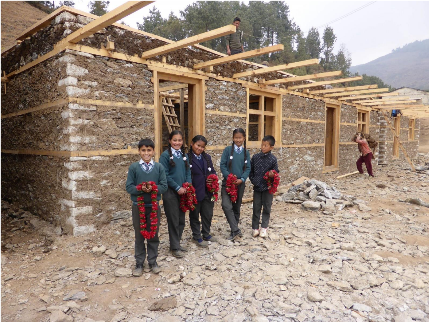
11 classrooms built with traditional, reinforced construction techniques
