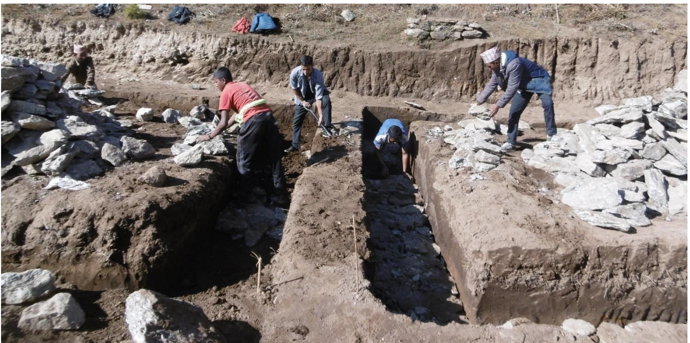
Foundations are done with big stones; all masonry work is done by hand
