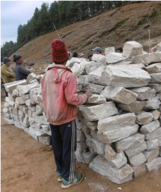
Corner stones and through stones are prepared and built properly for earthquake reinforcement
