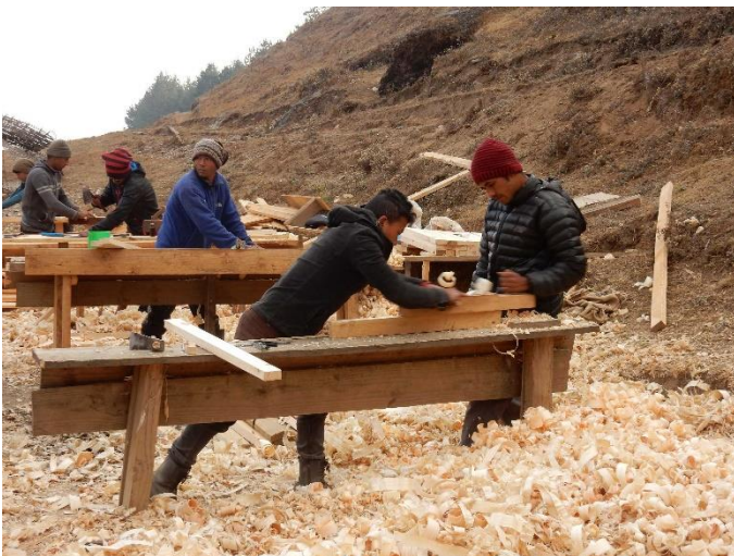
All carpentry work (door and window frames, ringbeams etc.) are done by hand. Paul explains details about the wooden earthquake reinforcements; they want to know
