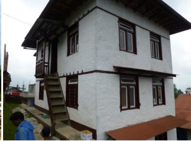
Ringbeam, big effect in holding walls together ! Several ringbeams for 2 storey building.
