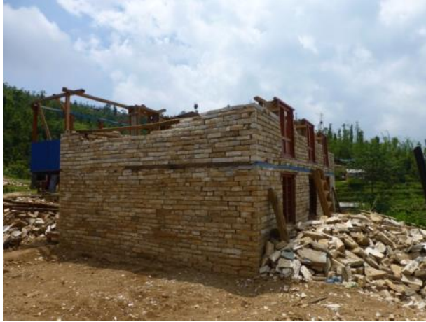
Ringbeam, big effect in holding walls together ! Several ringbeams for 2 storey building.
