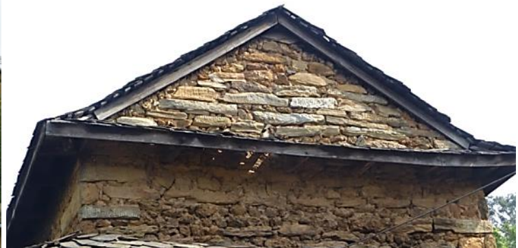
Gablewalls need to be bonded with roof construction ! Just a plank inside and outside of gablewall.
