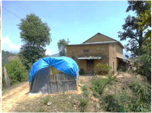
replacing emergency shelter
