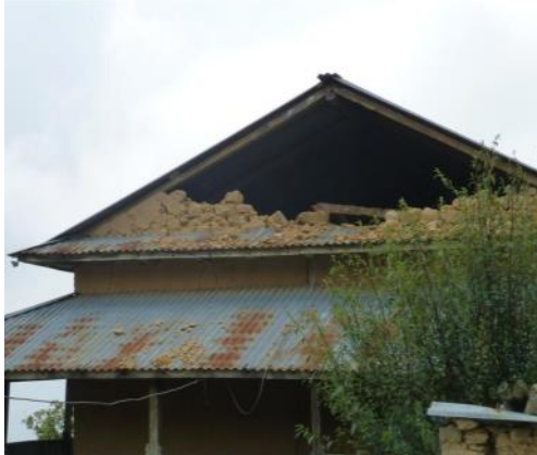
Gablewalls need to be bonded with roof construction ! Just a plank inside and outside of gablewall.
